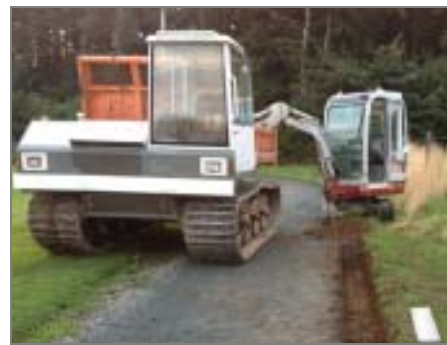
Improvement works 'on track' at Oxfield Community Park by Willie Regan Contractors.
