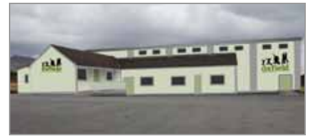
One of the colour schemes being considered for the re-painting of the Oxfield Community Centre.
