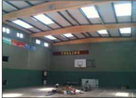
Skylights - A sneak preview of the new (and seriously bright!) roof at the Oxfield Centre
